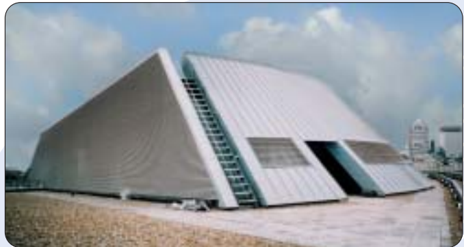
Custom Built Louvres for Land Securities Office Project.
