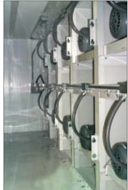
Vibration reduced due to reduction in airway tunnel turbulence.
