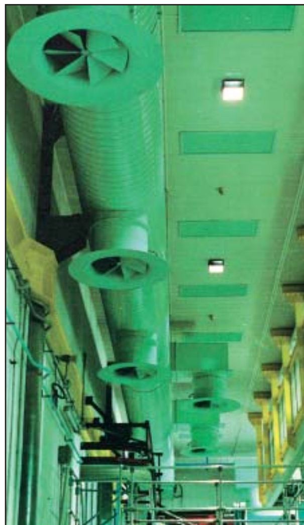
Installation of swirl diffusers in a printing office.
